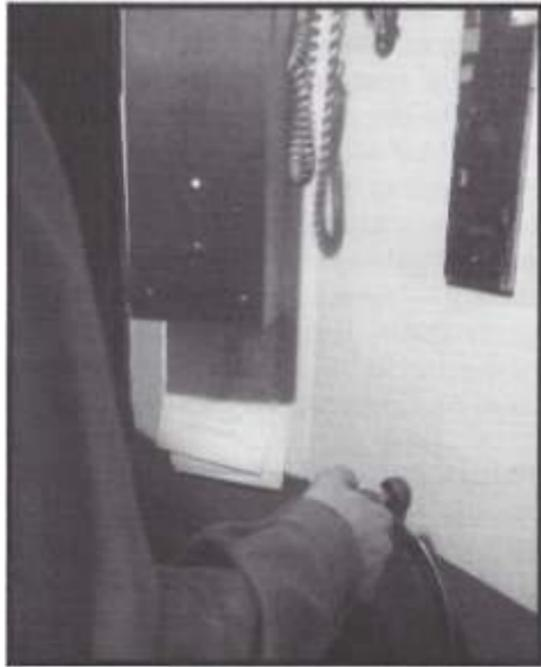
*Older, cooler elevators may lack up and down buttons and instead have one lever that controls speed and direction.*
