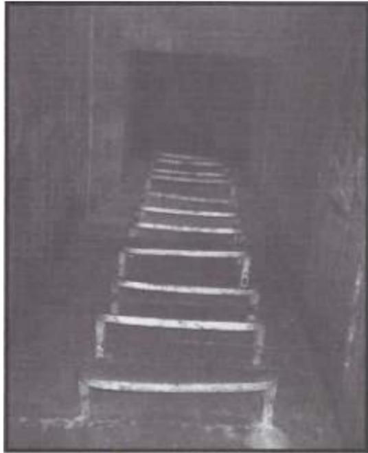
*Stepirons set into the concrete at the side of the drain are often used in place of ladders.*
